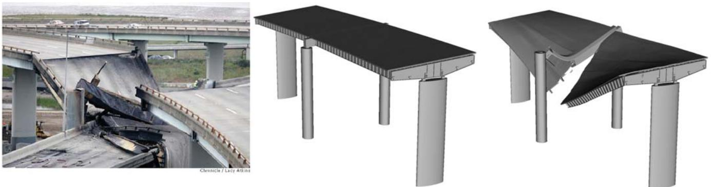
**Figure 3.** Simulated collapse of the MacArthur Maze connector using TOPAZ3D for the thermal loading and ParaDyn for the structural loading. (Photo courtesy of San Francisco Chronicle.)
